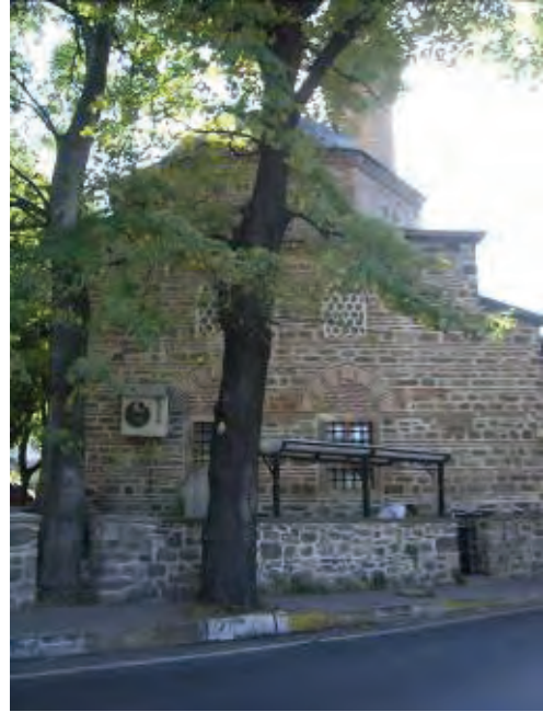
Bursa İmareti İsabey Cami arka cephe
